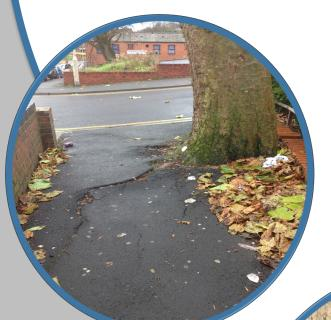
The issues with using traditional materials around tress are evident in the photos, left and below, where root growth and movement has had a severe impact on the footpath.
