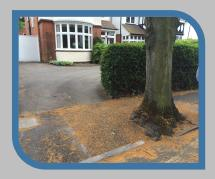
Above: With root intrusion spreading well beyond the normal tree pit boundary, Birmingham City Council engineers have now specified the use of KBI Flexipave into the wider pavement area.
