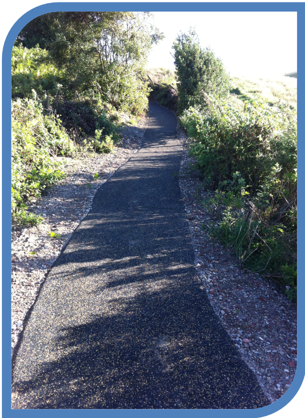
The finished bridleway conforms to the natural contours of the original path and is completely porous. The recycled rubber used within the material not only makes it eco-friendly, it reduces the impact on the leg joints of the horses using the bridleway.
