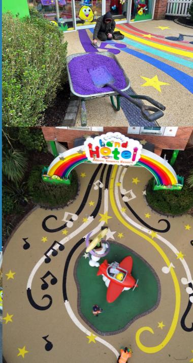
In order to do so, we removed all the existing surfacing and reprepared the groundworks and sub-base to make it fully permeable. We then installed our meadow Flexistone blend for the main area with six bespoke accompanying Colourbound colours, supplied by Vuba resin systems.
