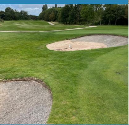
The image to the left shows the existing bunkers, with a concrete based liner. The main issue with this system is the sand can migrate from the bunker faces.
